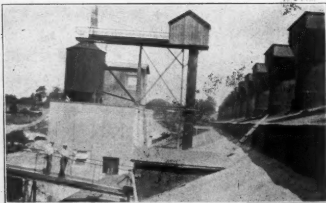
Hydrating Plant and Kilns
